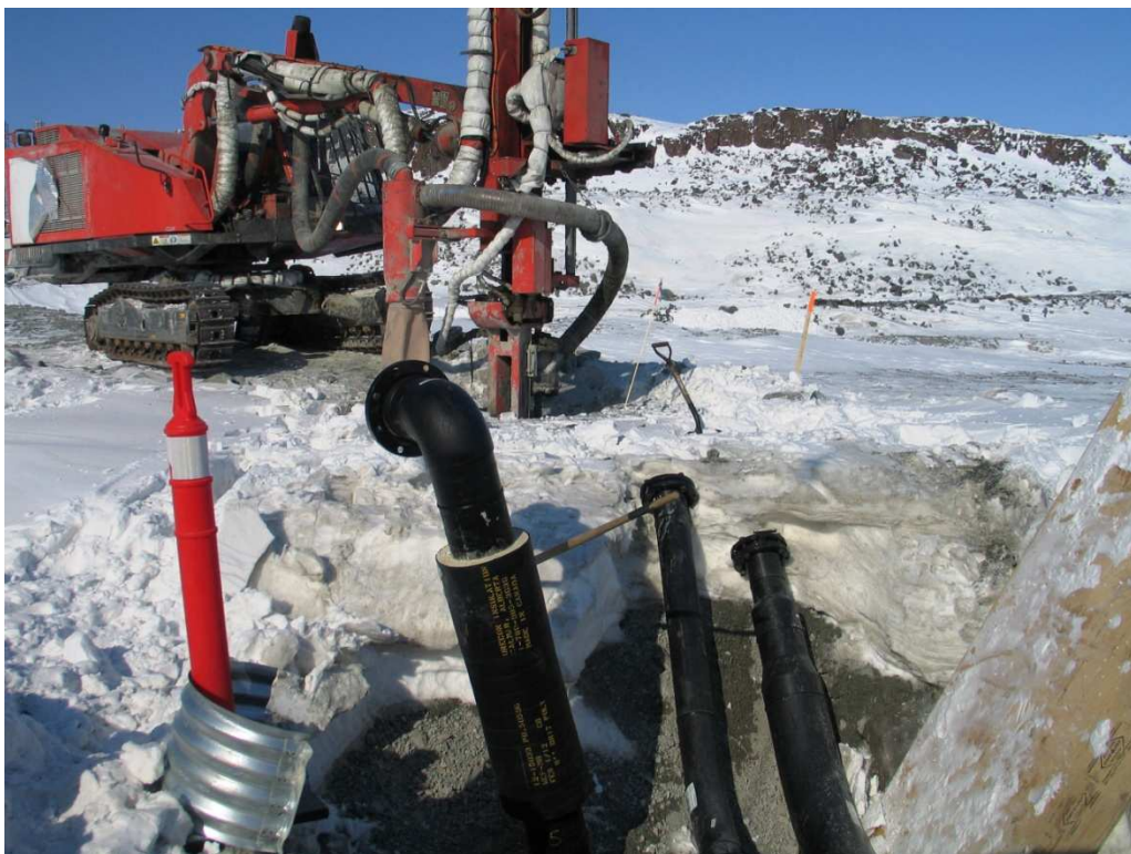
Photo 6: Drilling thermister SRK-GTC-DH01 between the Sedimentation Pond and Pollution Control Pond. Note proximity to pipes for pumping the pollution pond.
