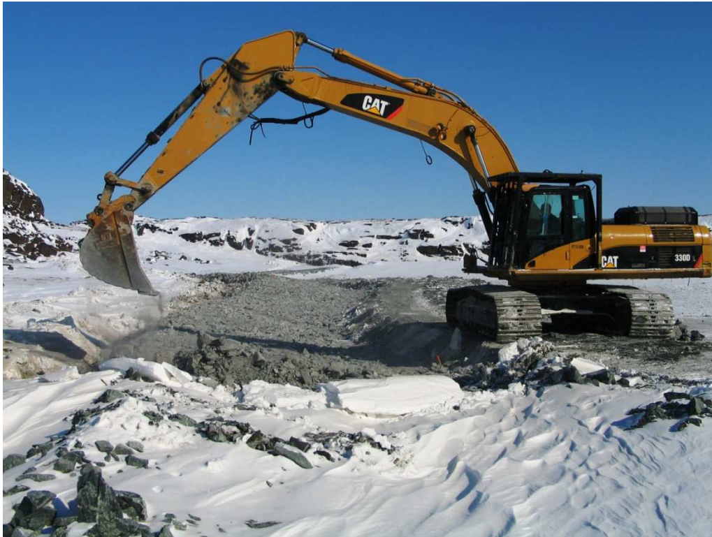
Photo 3: Placing second lift of ROQ. Connecting to previously placed ROQ ~Sta 4+00
