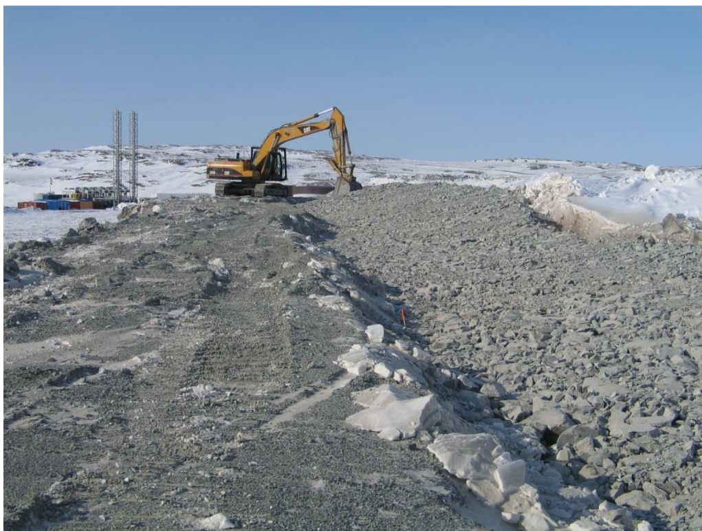
Photo 1: Placing ROQ ~ Sta 4+50 at start of shift.
