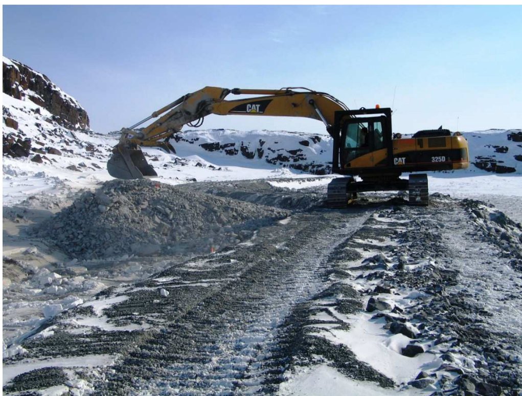
Photo 1: Placing ROQ ~ Sta 4+50 at start of shift.
